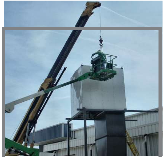
Installation of a weather covered separator
