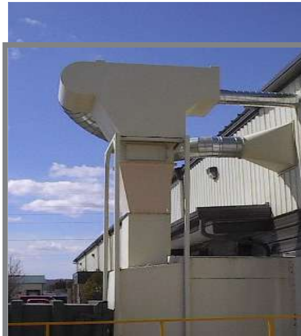
Separator with a return air system and discharge chute into a compactor
